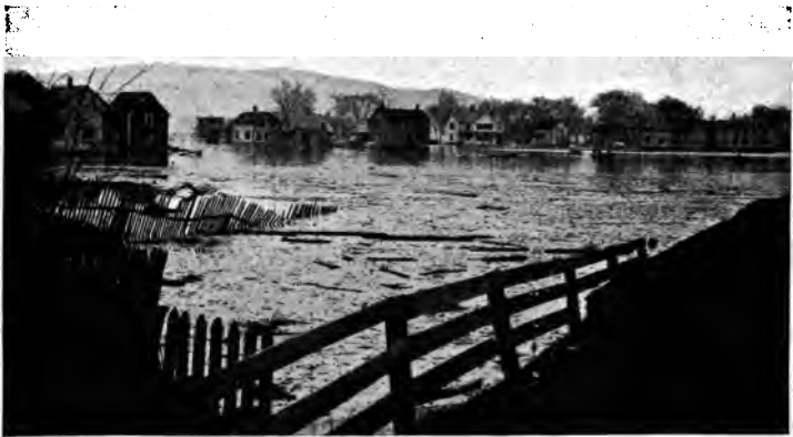
High water on the outskirts of Northampton
